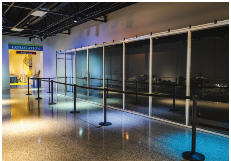
A newly constructed controllable micro-climate case, based on the design of a clean room, stands outside of the Exploration Gallery. The case will be filled with objects after undergoing environmental testing.
